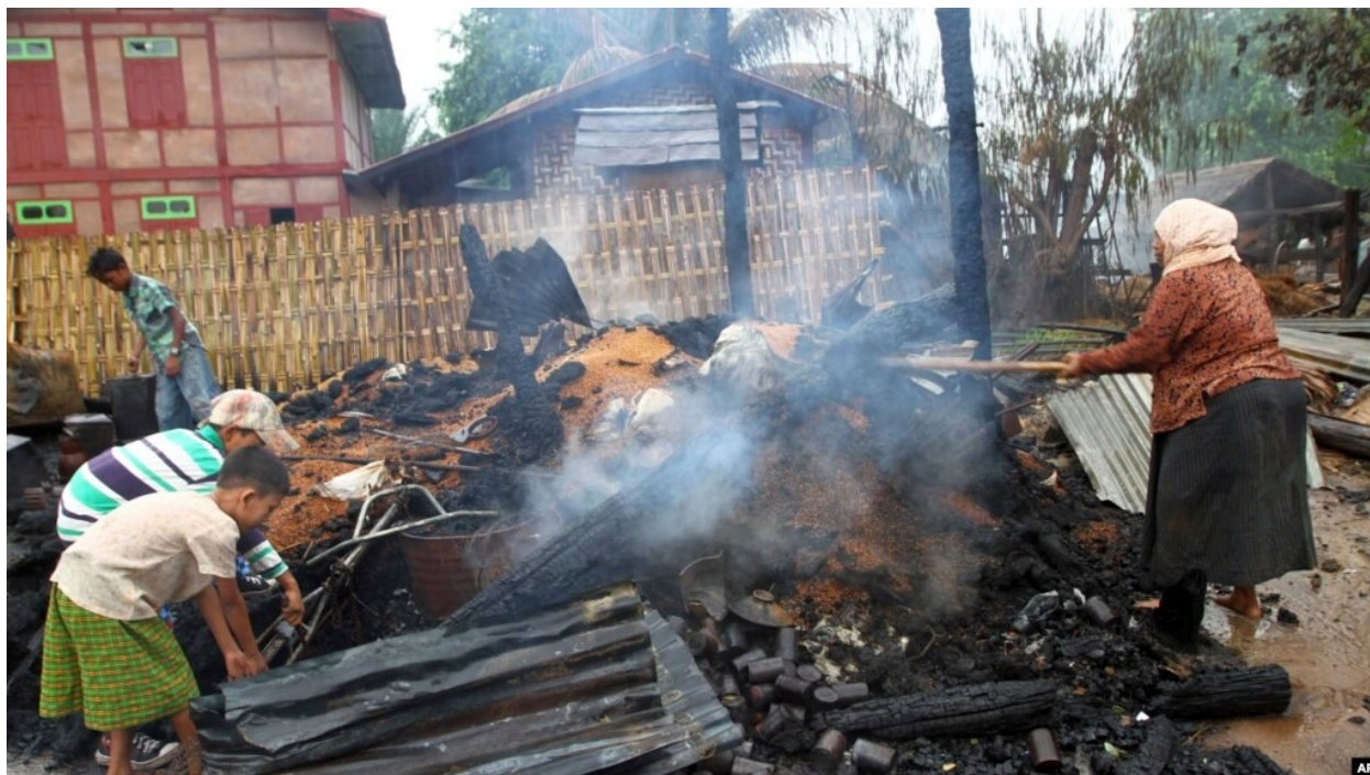
A Muslim woman and children clear debris of a burnt-down building in Htan Gone village of Kantbalu township, Sagaing Division, Burma, Aug. 26, 2013. (Photo: AP)
